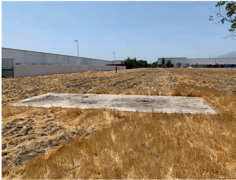
Photo #9 View of concrete residential building foundations located in southeastern portion of the Property. View looking to the west.
